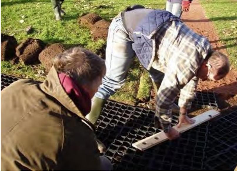
The EcoGrid reinforced pathways mean complete access routes are now available for wheelchairs - no churning up mud, no unsafe conditions - all done quickly with minimal cost and labour.
