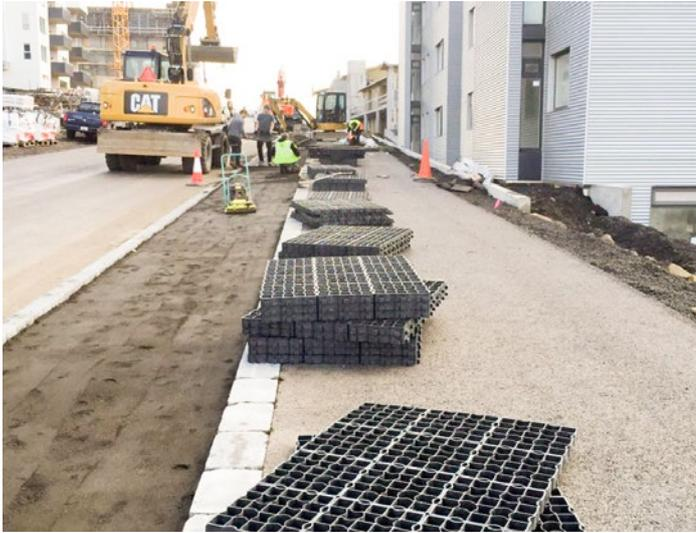
Here the client required a free draining, natural overspill parking area in a busy city centre. Time and maintenance were an issue in the short term as they required an 'instant' grassed effect, not being able to seed the area, water and wait for the seed to germinate.
