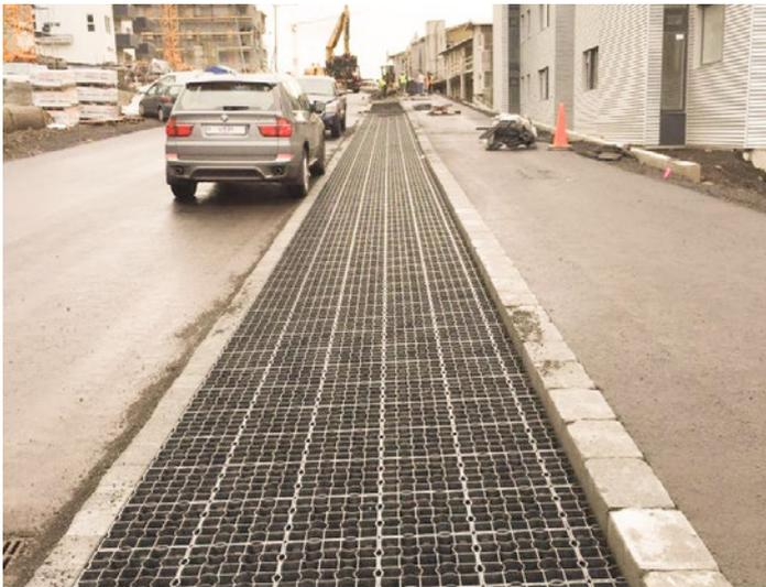
The grids were then laid in a very short time. This is possible because EcoGrid comes in pre-locked sheets of 12 grids or 1.33 square metres. Important when you consider other grids need to be laid individually and often require separate pins or clips. The grids were then 80% filled with topsoil.
